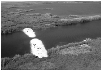
Oil-drilling access canal plug.
